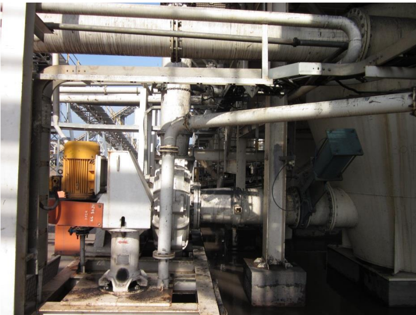
ELM-350S in Coal Washery in Indonesia
